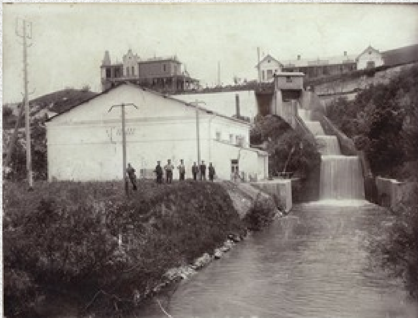
Belyi Ugol' hydroelectric power station
